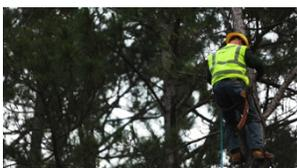
When aloft with hand saws, cover the cutting teeth when not in use.
