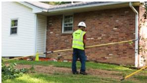
Downed and energized conductors or energized objects present the hazard of step potential and electric shock.
