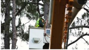
Simultaneous contact with two separate energized conductors is phase-to-phase contact. Direct or indirect contact with an electrical conductor, energized tree limb or other energized object is phase-to-ground contact.
