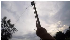
Locate and identify electrical hazards in or near the tree. Maintaining the minimum approach distance (or MAD) is one of our Keys to Life.
